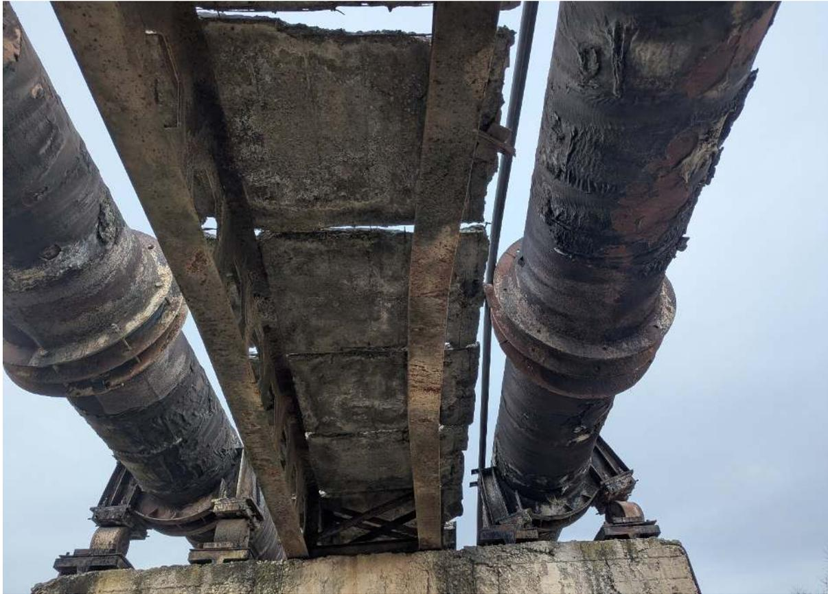
*Fig. 10. Deformed beam of the lower side 10th span*
