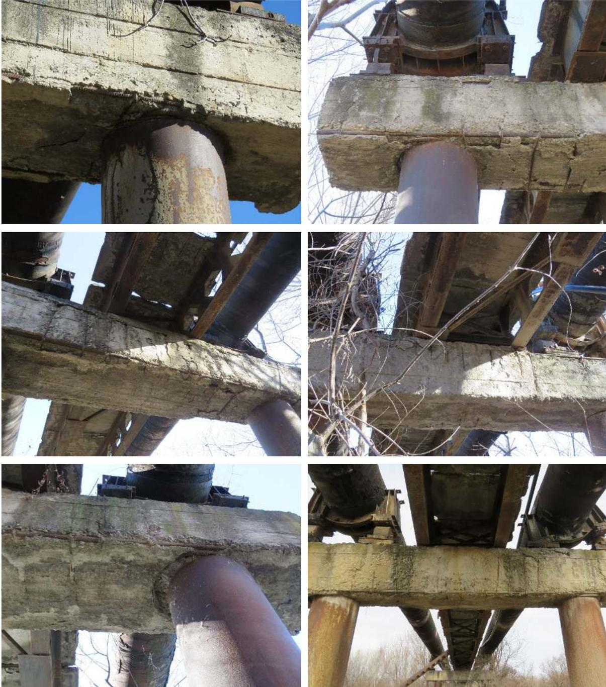
*Fig. 1. Damaged protective layer concrete of reinforced concrete crossbar*
