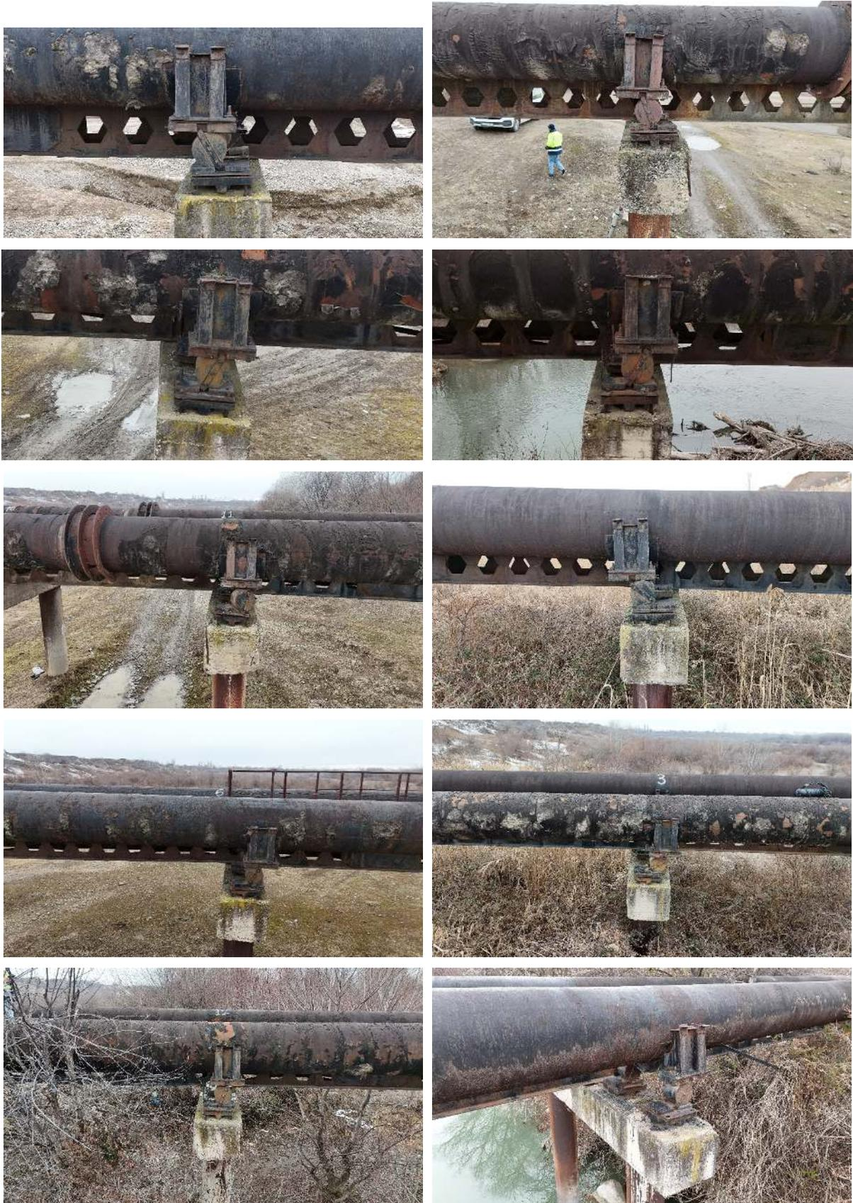
*Fig. 6. Bearing roller falling out of the balance sheets*
