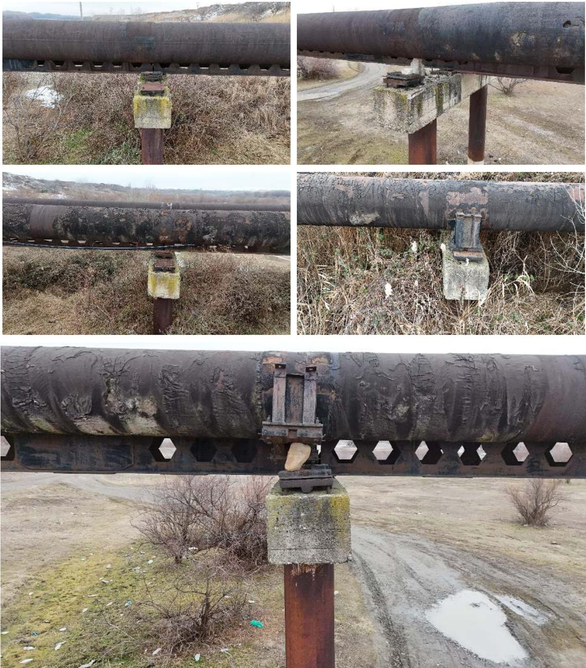
*Fig. 4. Support parts without rollers*
