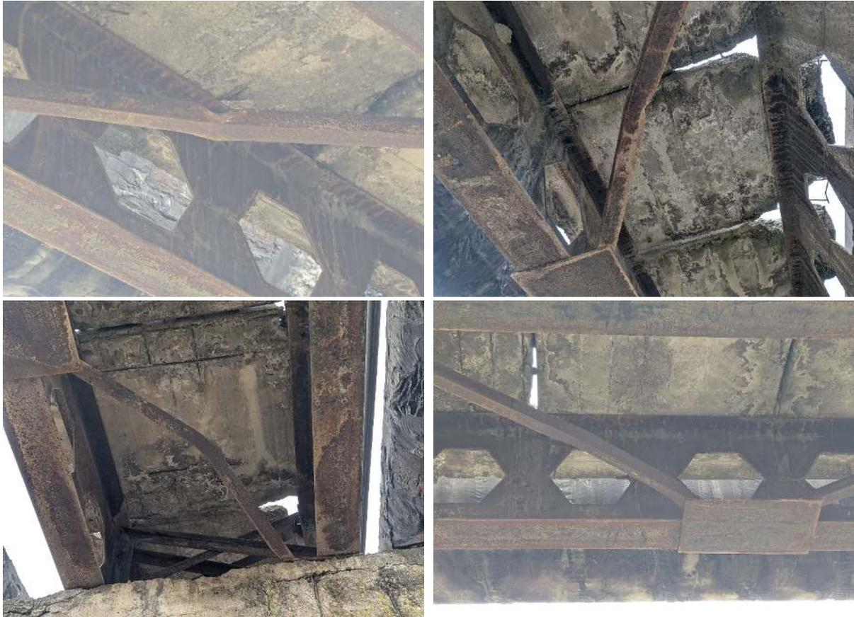
*Fig. 8. Deformed longitudinal connections*
