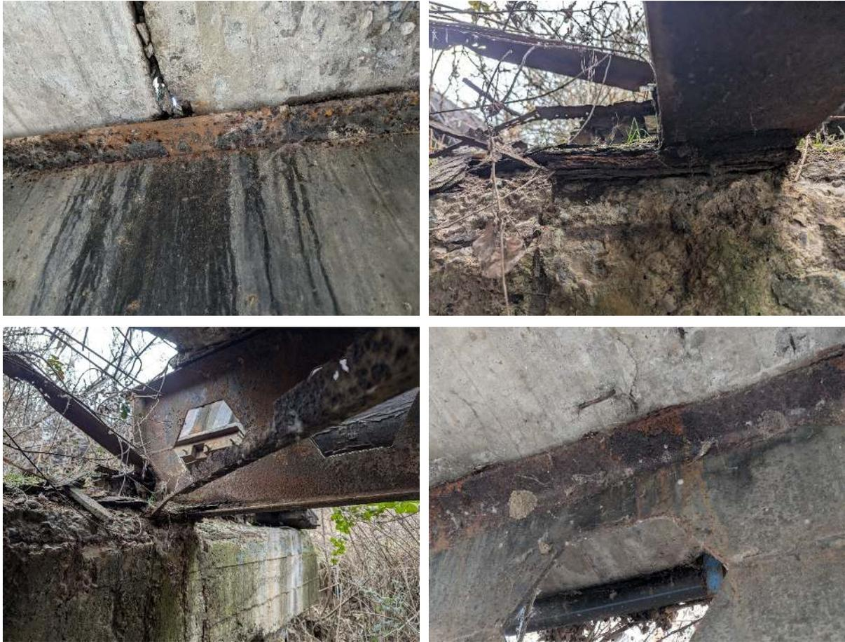
*Fig. 7. Rusted steel elements of the span*
