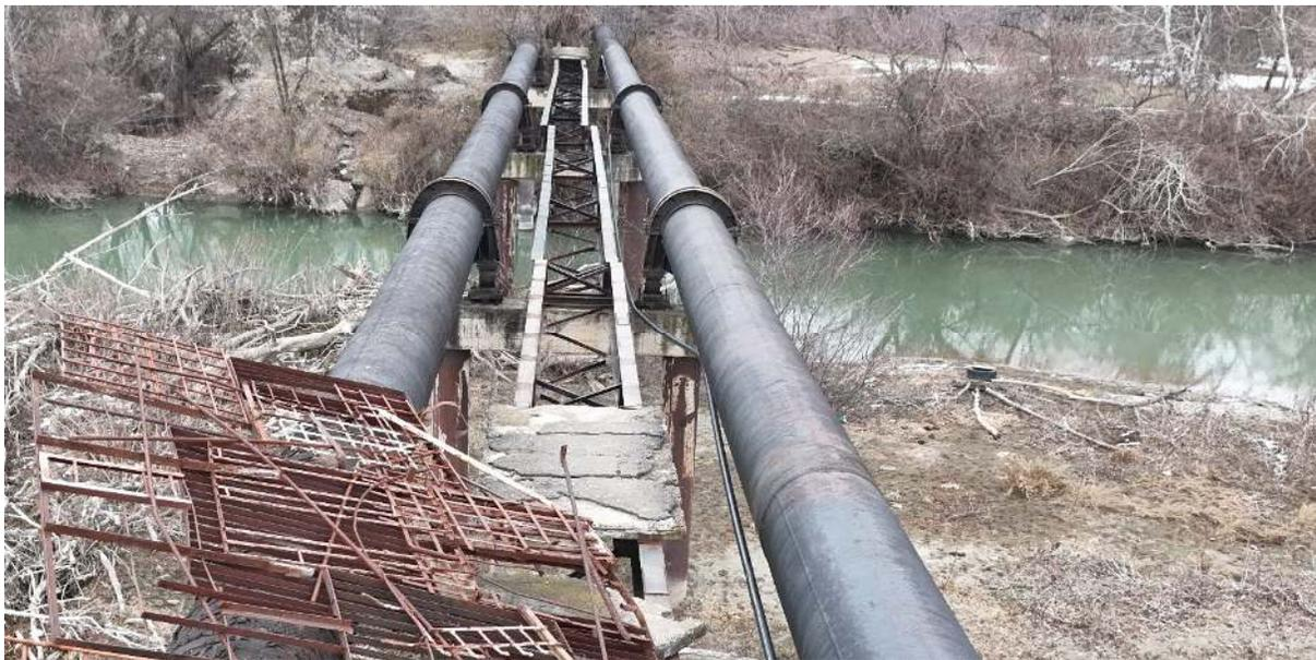
*Fig. 11. Arrangement of longitudinal beams in N29 and N30 span*
