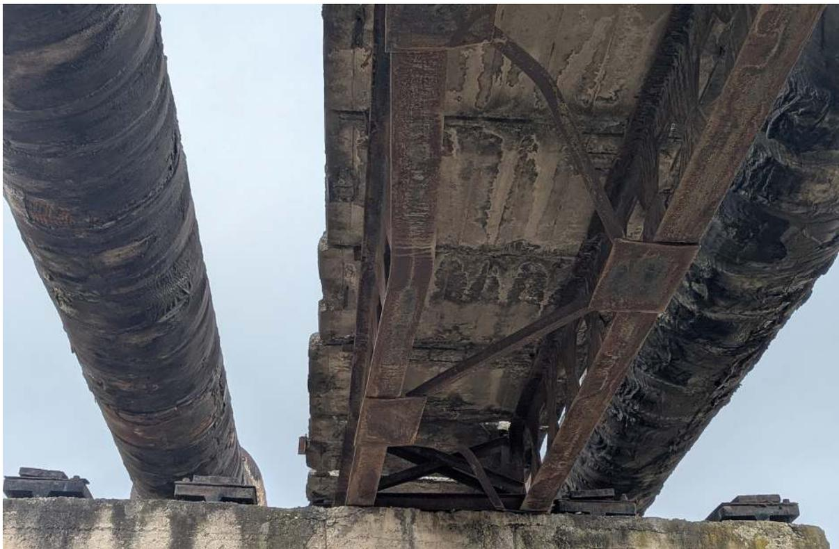
*Fig. 9. Deformed beam of the upper side 9th span*
