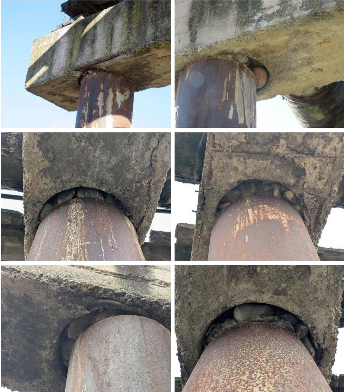
*Fig. 2. View of the connection node between the reinforced concrete crossbar and the steel post*
