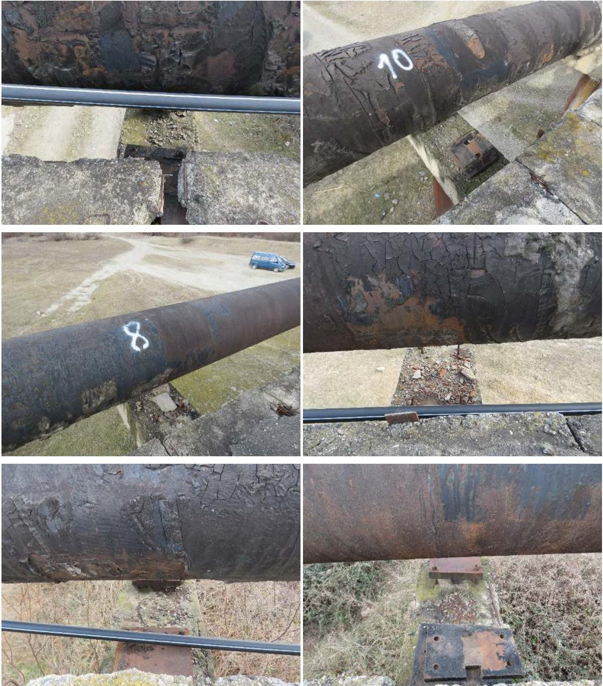
*Fig. 3. Water pipe without supporting parts*
