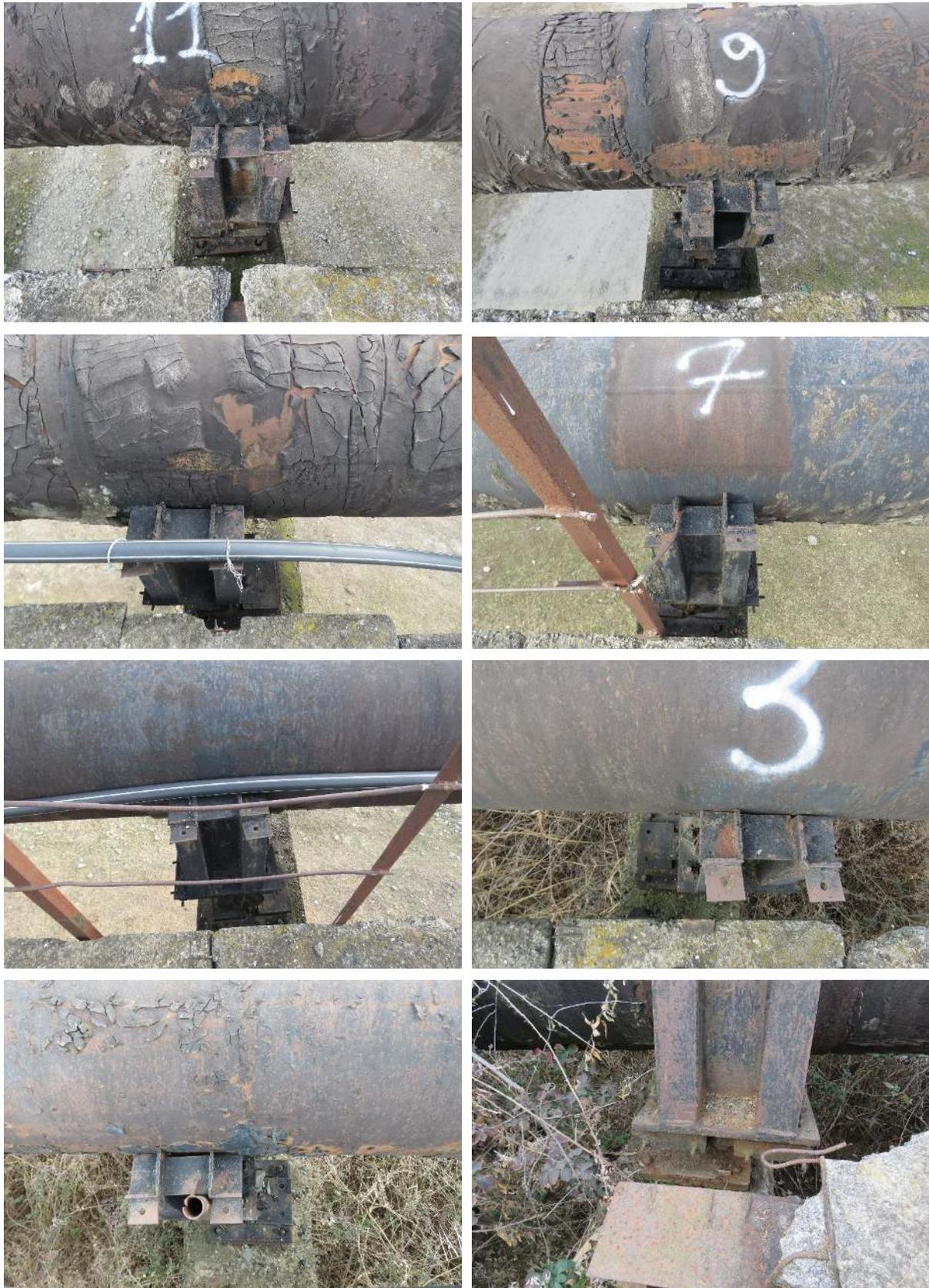
*Fig. 5. View of the steel support structures of the water pipeline*
